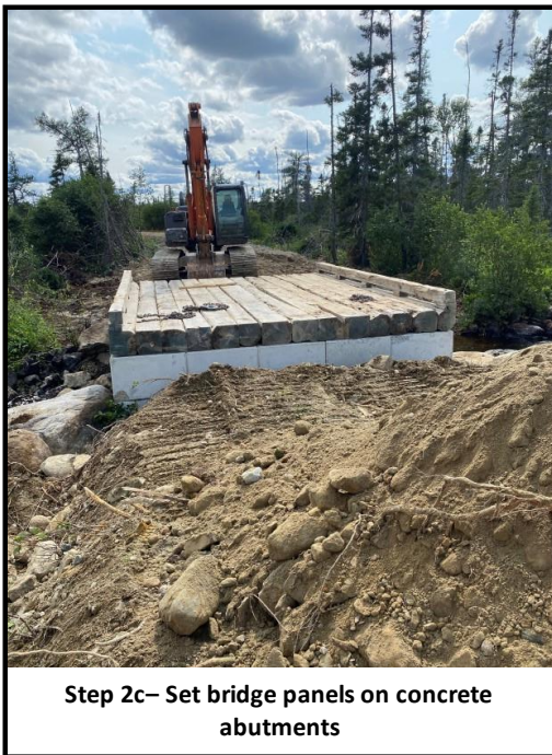
Plate 4-3 Example of bridge materials and building methods utilized on permitted upgrades to the main Atlantic Lake Forest Access Road.
