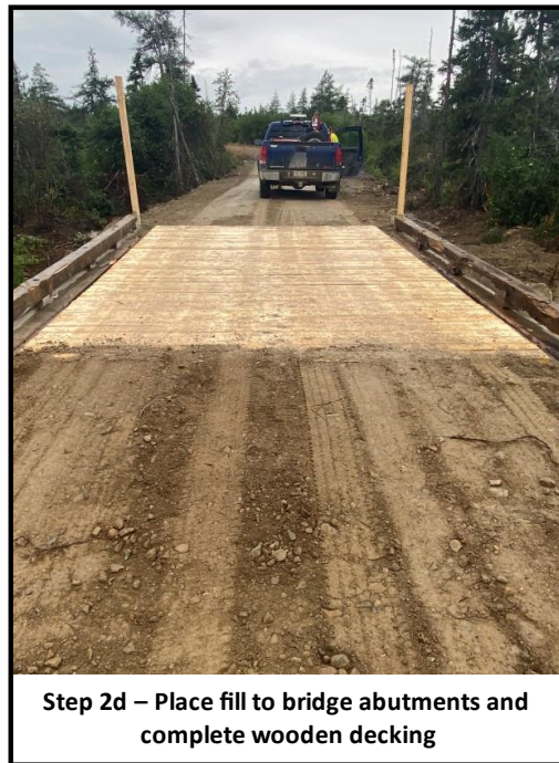
Plate 4-3 Example of bridge materials and building methods utilized on permitted upgrades to the main Atlantic Lake Forest Access Road.
